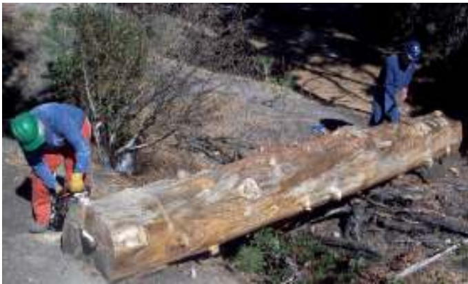
John McKenna (with chain saw) and Phil Brisack start shaping the log bridge
