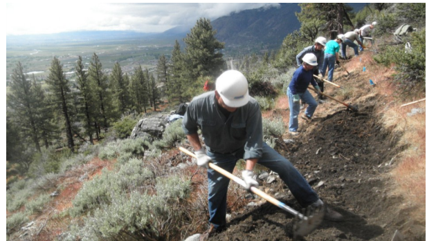
Volunteers working on the Genoa area trails project
